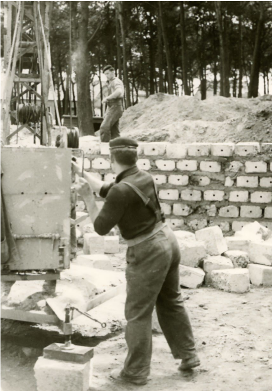
One of the photographs taken by the architect, Mathieu Driessen, during his regular visits to the building site of the CCI, ca 1961. Source: KADOC-KU Leuven.
