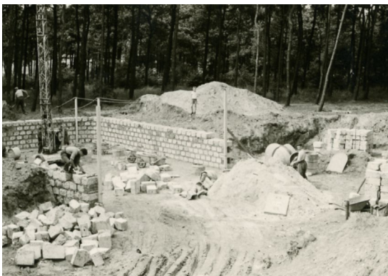
Construction site of the Centro Cattolico Italiano (CCI) in the mining town of Waterschei. Photograph taken by the architect of the building Mathieu Driessen, Belgium, ca 1961. Source: KADOC-KU Leuven
